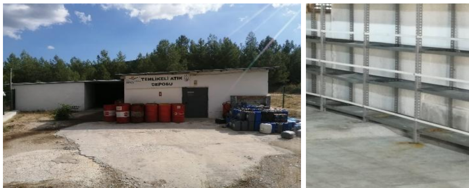
Figure 12: Hazardous Waste Warehouse
